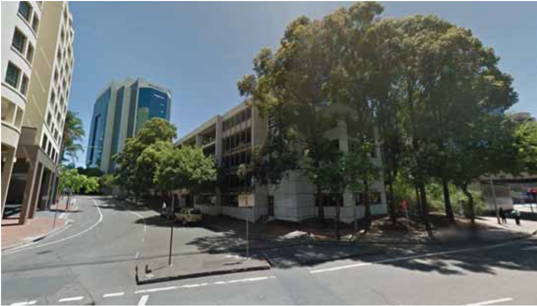
EXISTING CARPARK BUILDING
