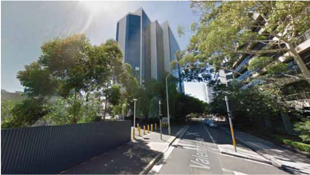
EXISTING OFFICE TOWER
